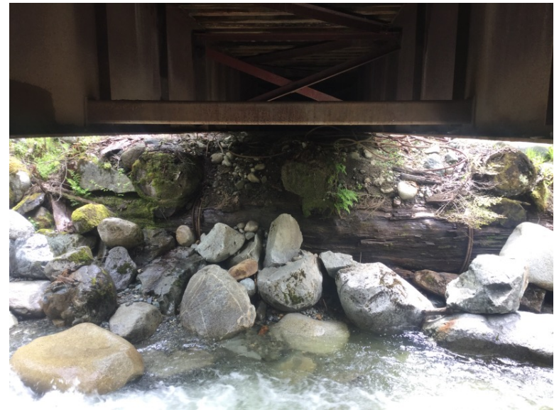
Left Bank Abutment when facing downstream
