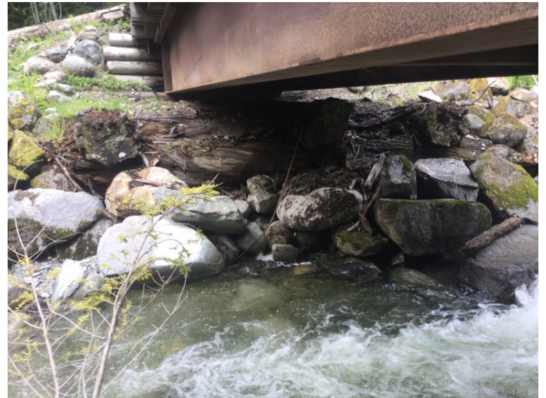
Right Bank Abutment when facing downstream
